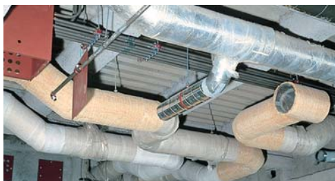
Thermal Insulation Materials Rock wool and glass wool for use in residential, office building and plant construction
